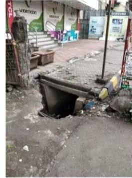
Lined, covered drains
