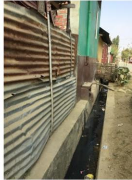
Lined, open drains
